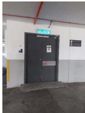
**Figure 4.** Steep ramp in front of entrance in multi-level parking in CS1
