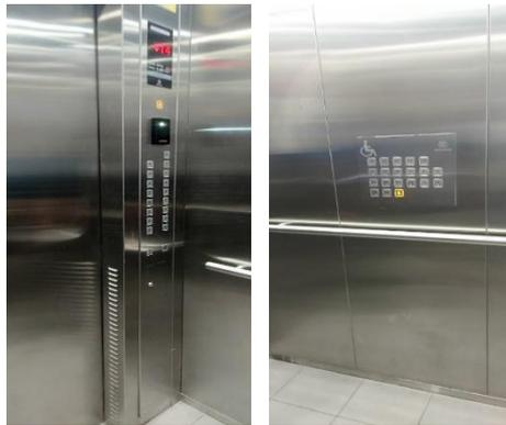
**Figure 5.** Vertical button panel for typical users (left); horizontal button panel for the lower-reach users (right)
