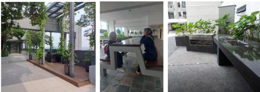
**Figure 8.** Wooden decking lacks of ramp in CS1; impractical bench and table height in CS2; insufficient knee clearance for the hand basin, and the faucet handle is beyond reach in CS3 (from left to right)
