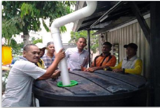
Figure 6: RA2's installation of rainwater harvesting system.
