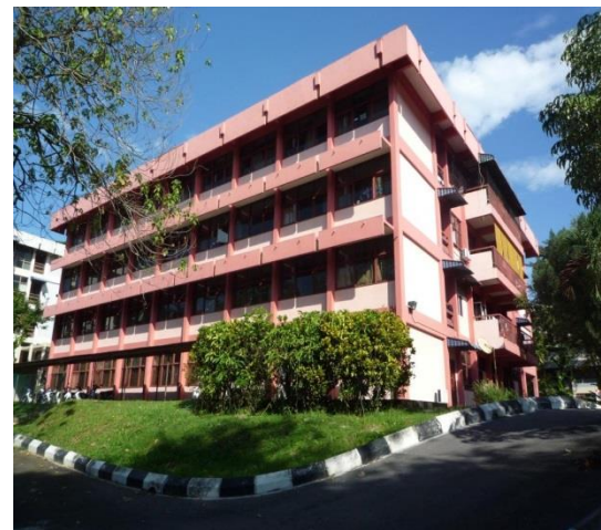
(a) Built-form configuration, enclosure and facade design - Large horizontal overhangs along the wall with windows
