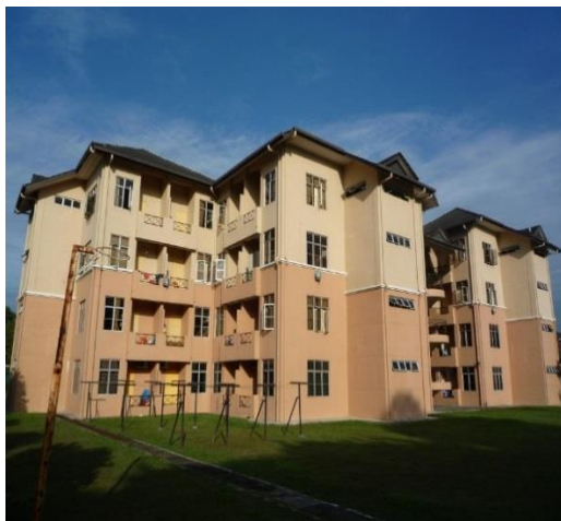
(a) Built-form configuration, enclosure and facade design - Large horizontal overhangs along the wall with windows
