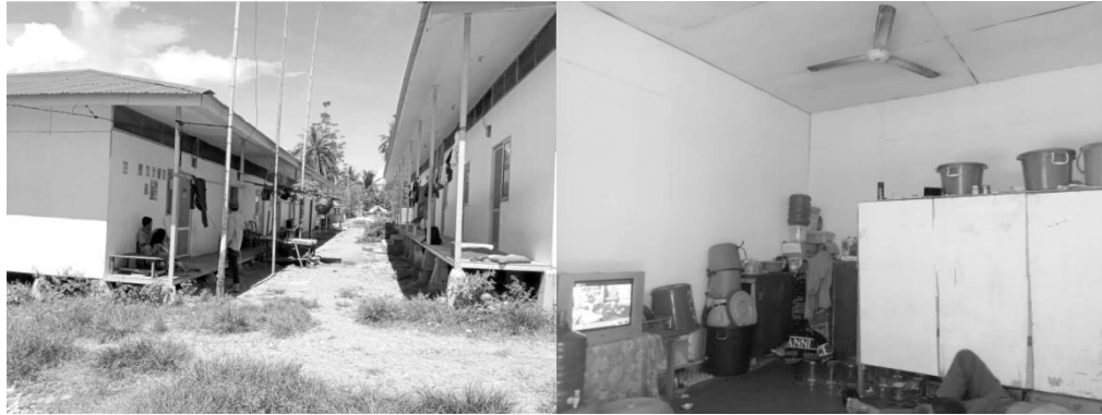
Figure 7. PUPR shelters by shared houses with lightweight structures and calcium board lay on concrete poles
