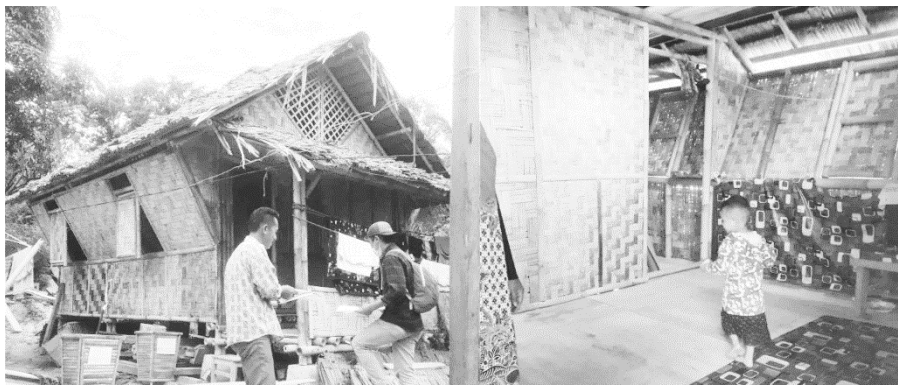
Figure 5. KUN shelters distinguished by bamboo structure and multiplex floor on a wooden stilt
