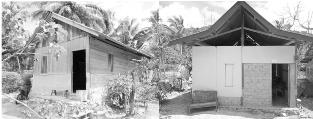
Figure 1. CRS shelters type by wood frame combined with wooden and brick wall on the ground
