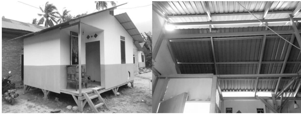
Figure 3. HABITAT shelters lightweight structure with metal materials on the wooden frame stilt
