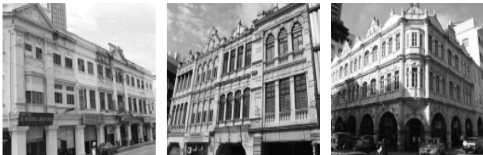
Fig2. Building façades in the study area
