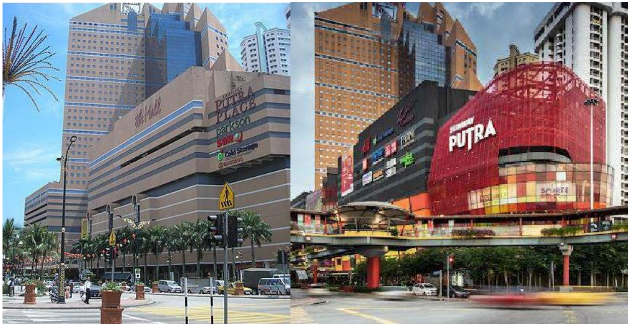
Figure 5. Before (left) and After (right) comparison photo of The Mall that was built in 1987 and underwent façade retrofit into Sunway Putra Mall in 2015
